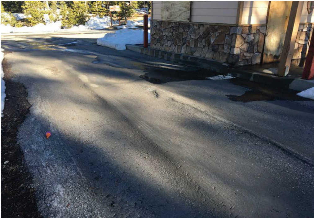
Photograph 1. Severe rutting at station 0+00. View looking north.
