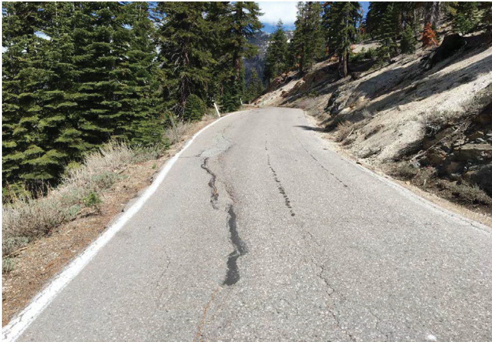
Photograph 3. Moderate severity longitudinal cracking at station 84+50 View looking northeast.
