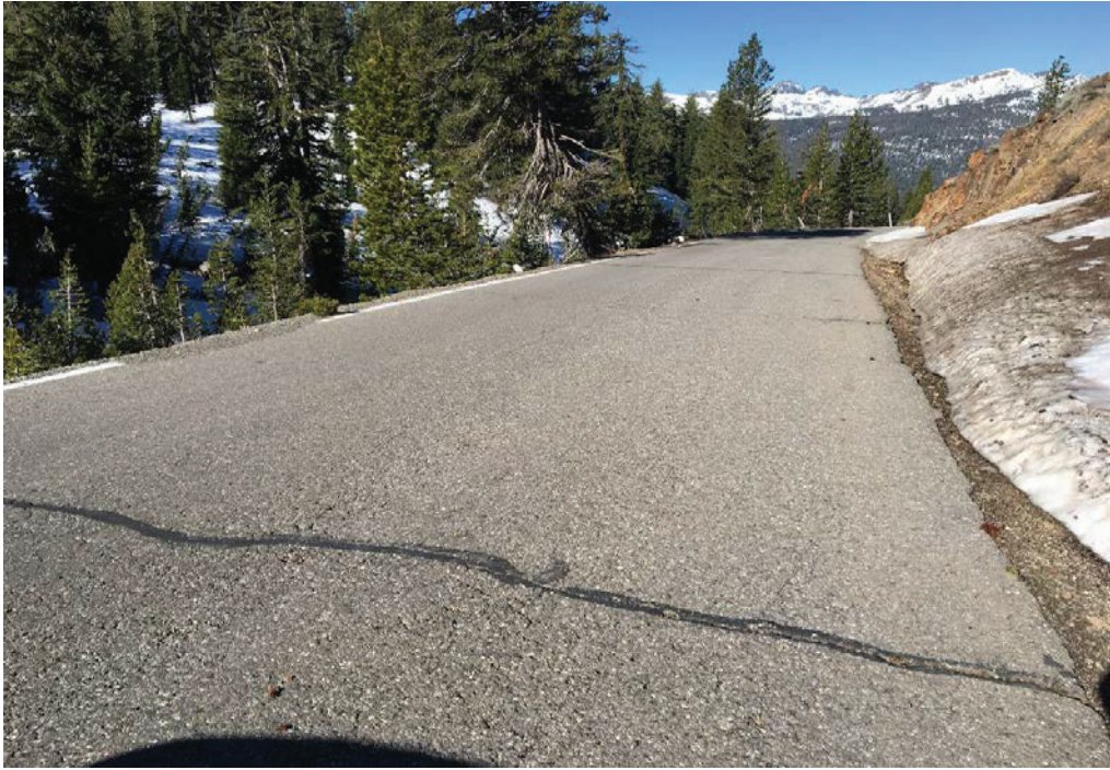
Photograph 5. Moderate severity transverse cracking at station 13+50. View looking southwest.
