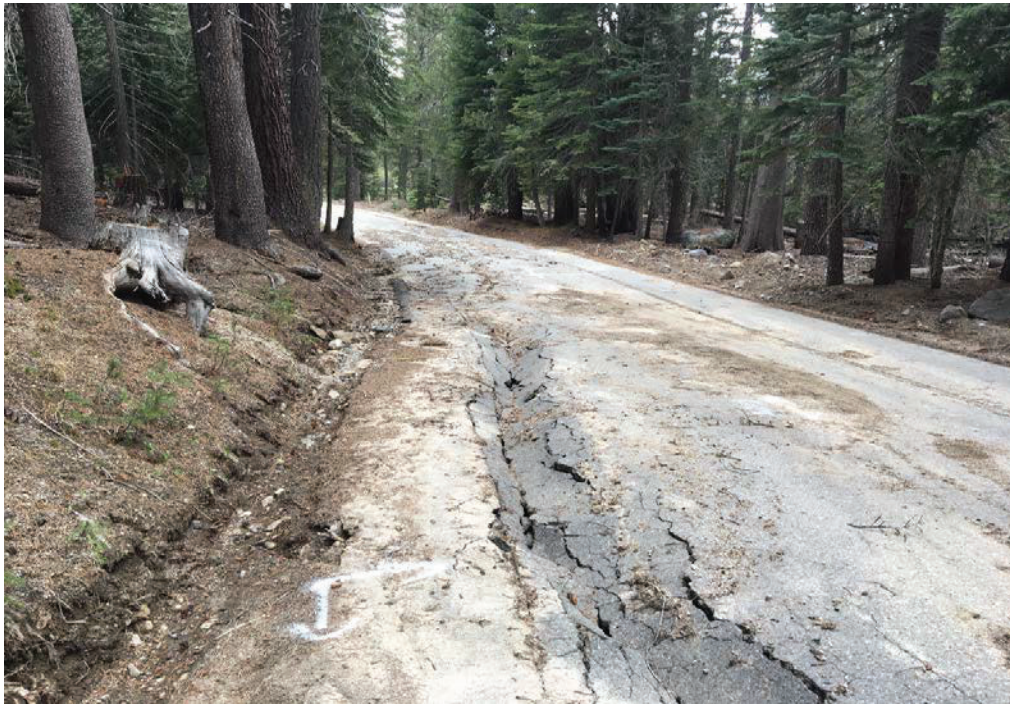
Photograph 2. Severe rutting at station 758+00. View looking west.
