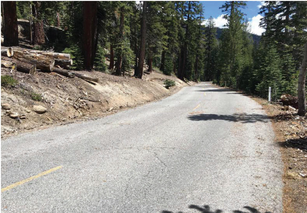
Photograph 6. Low severity fatigue cracking and rutting at station 358+00. View looking south.
