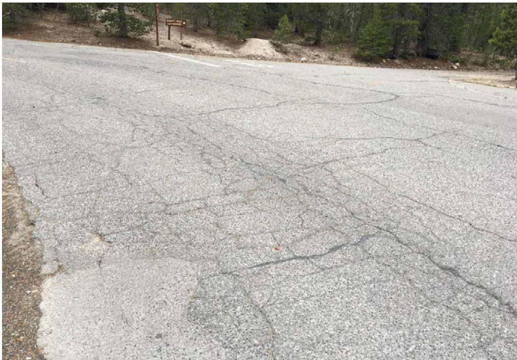
Photograph 4. Moderate to high severity block and fatigue cracking at station 685+00. View looking west.
