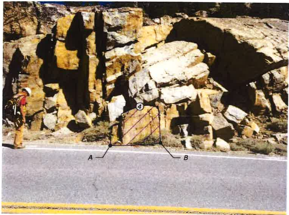
ROCK CUT LIMITS Station 314+09 to 314+20
