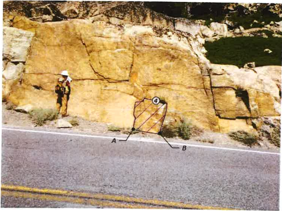
ROCK CUT LIMITS Station 318+27
