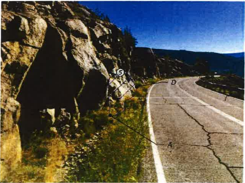
ROCK CUT LIMITS Looking Upstation Station 311+00 to 311+45
