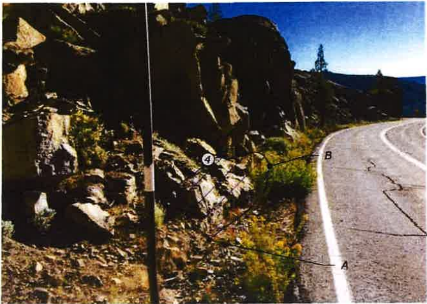
ROCK CUT LIMITS Looking Upstation Station 311+85 to 311+95
