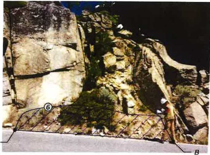
ROCK CUT LIMITS Station 325+00 to 325+25
