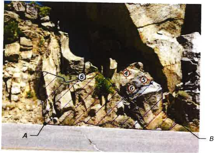
ROCK CUT LIMITS Station 325+25 to 325+50
