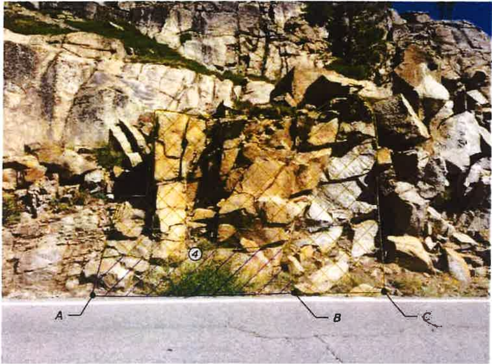
ROCK CUT LIMITS Station 311+85 to 311+95
