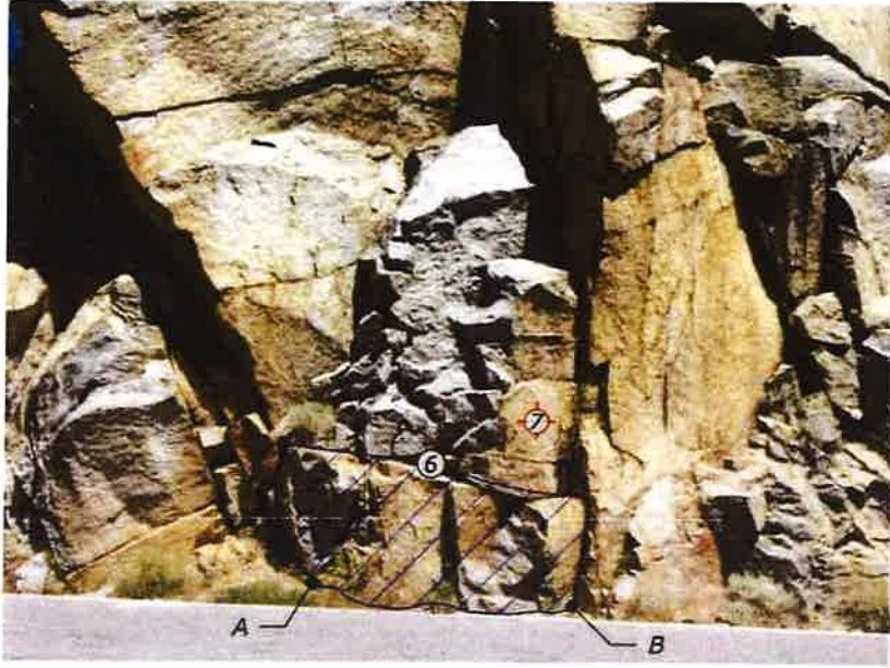
ROCK CUT LIMITS Station 325+50 to 325+65
