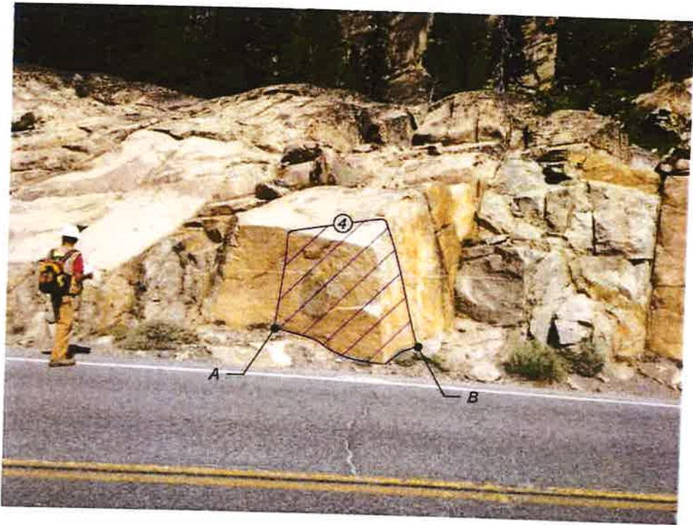
ROCK CUT LIMITS Station 317+85 to 317+95
