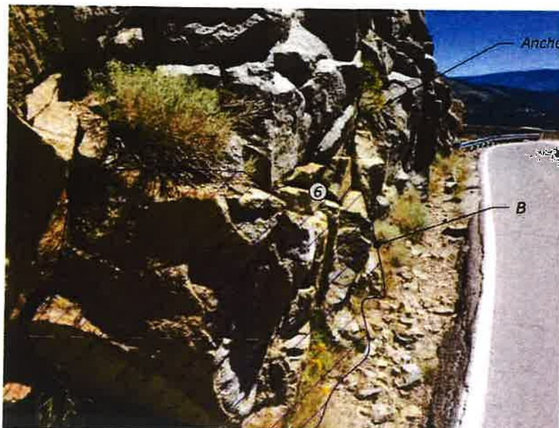
ROCK CUT LIMITS Looking Downstation Station 325+50 to 325+65
