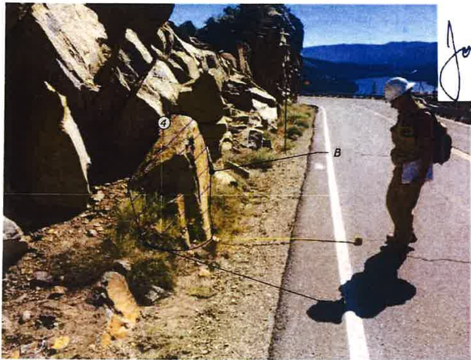
ROCK CUT LIMITS Looking Upstation Station 314+09 to 314+20
