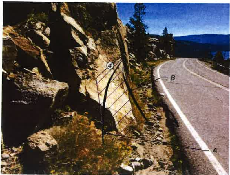
ROCK CUT LIMITS Looking Upstation Station 312+30 to 312+36
