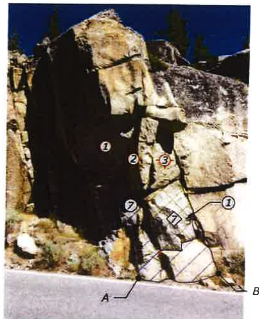
ROCK CUT LIMITS Station 324+88 to 325+00
