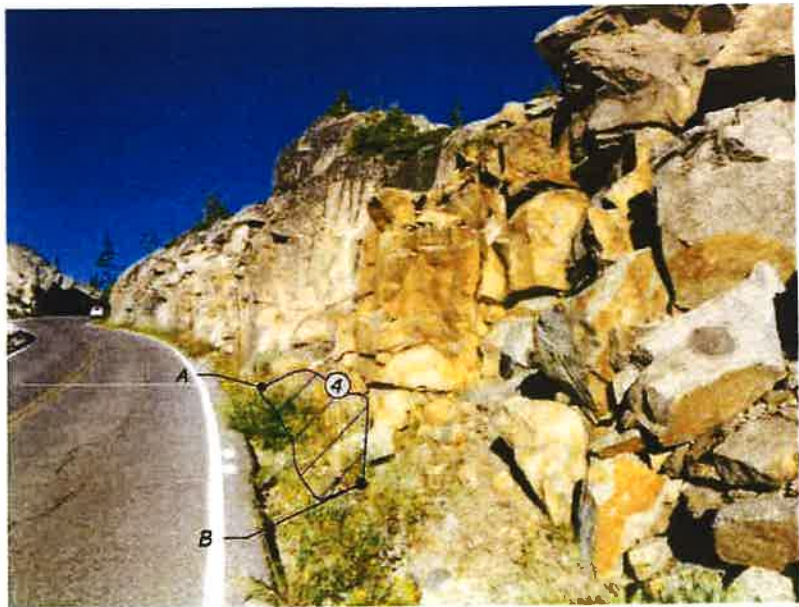
ROCK CUT LIMITS Looking Downstation Station 311+85 to 311+95
