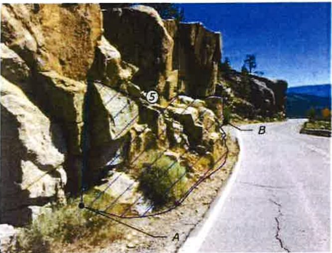
ROCK CUT LIMITS Looking Upstation Station 322+00 to 322+50
