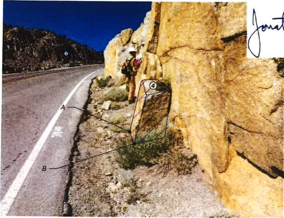
ROCK CUT LIMITS Looking Downstation Station 318+27
