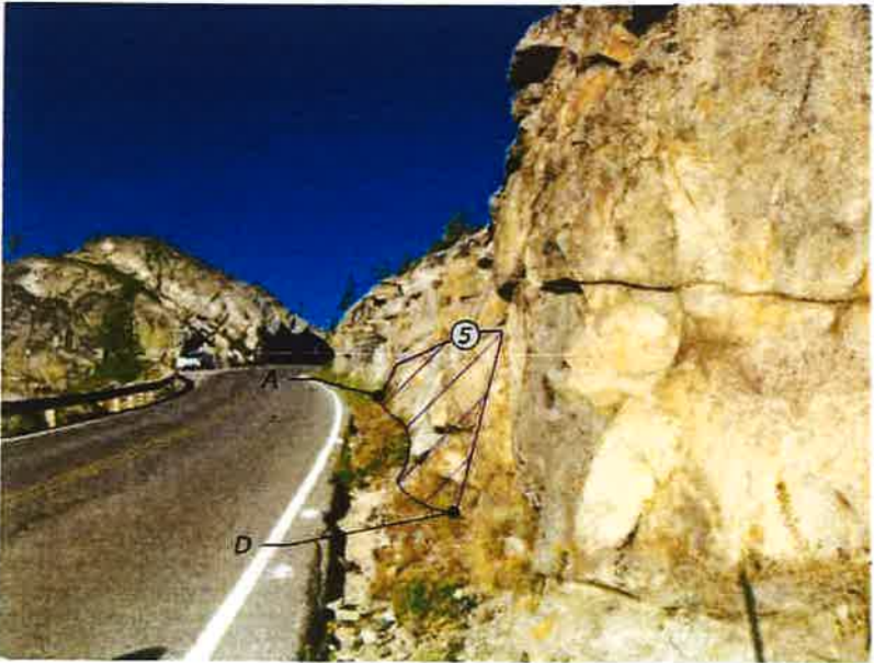
ROCK CUT LIMITS Looking Downstation Station 311+00 to 311+45
