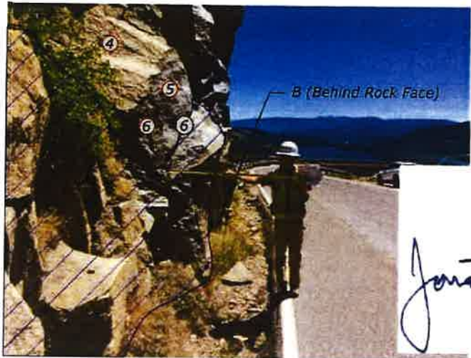
ROCK CUT LIMITS Looking Upstation Station 325+25 to 325+50
