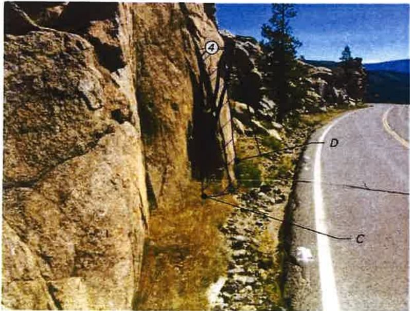
ROCK CUT LIMITS Looking Upstation Station 312+30 to 312+36
