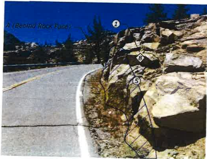
ROCK CUT LIMITS Looking Downstation Station 366+35 to 366+90
