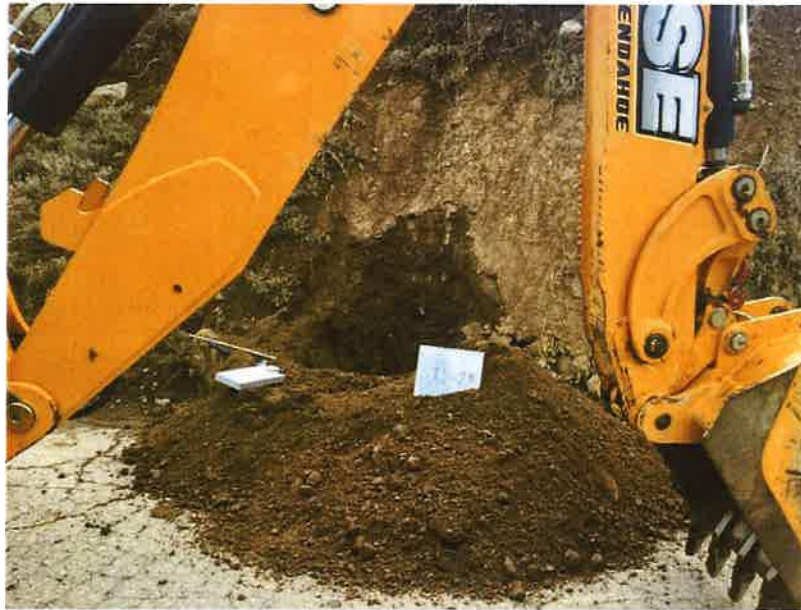
Photograph 45. Test Pit TP-2 during excavation.
