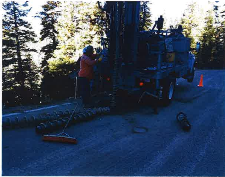
Photograph 55. Boring SW-B-47 during drilling.
