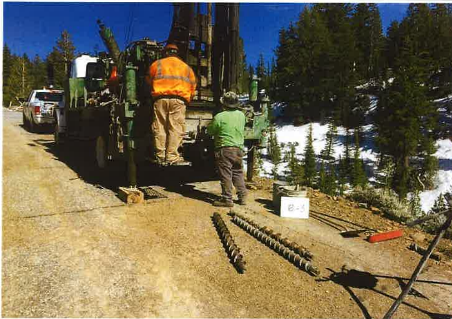
Photograph 3. Boring SW-B-03 during drilling.
