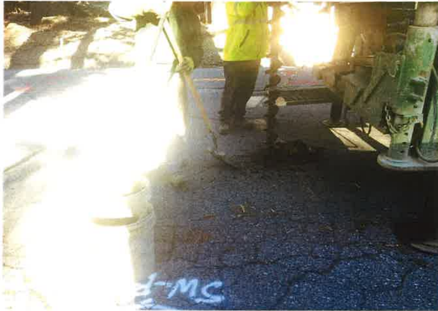
Photograph 39. Boring SW-B-39 during drilling.
