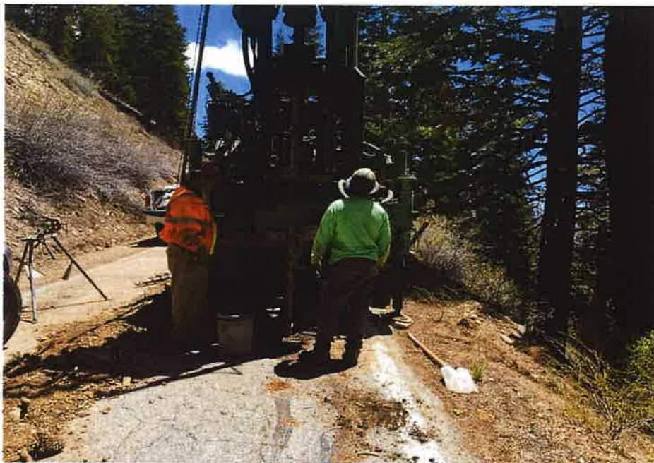
Photograph 6. Boring SW-B-06 during drilling.
