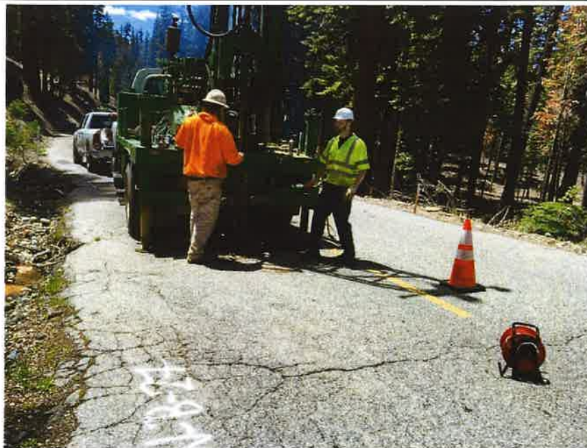
Photograph 27. Boring SW-B-27 during drilling.
