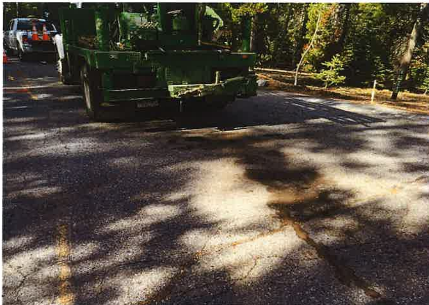
Photograph 32. Boring SW-B-32 during drilling.
