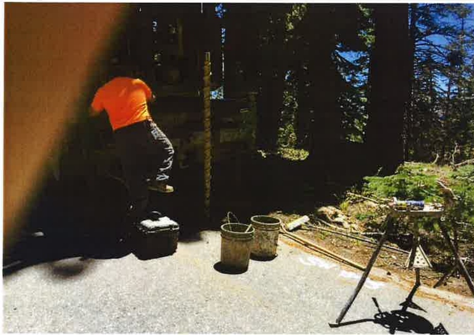
Photograph 13. Boring SW-B-13 during drilling.
