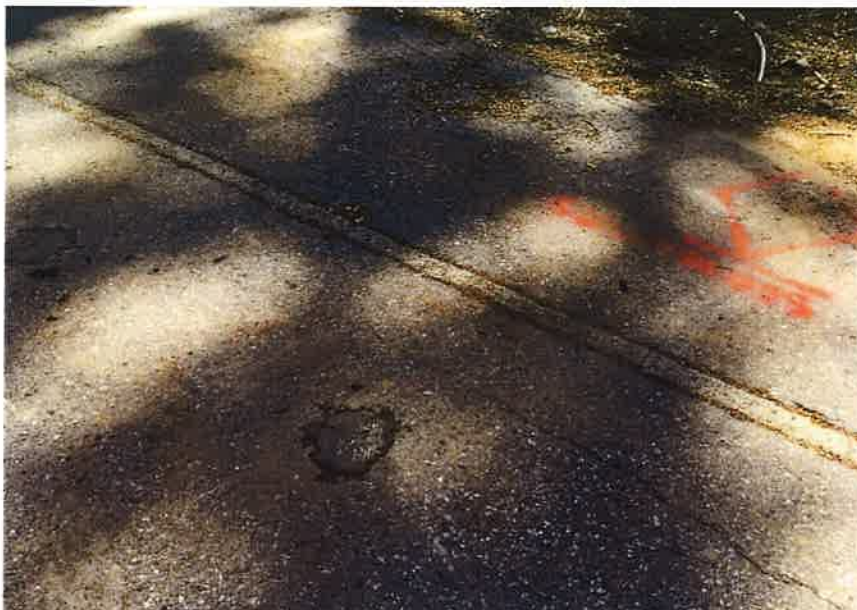
Photograph 40. Boring SW-B-40 after drilling.
