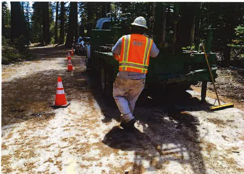
Photograph 30. Boring SW-B-30 during drilling.
