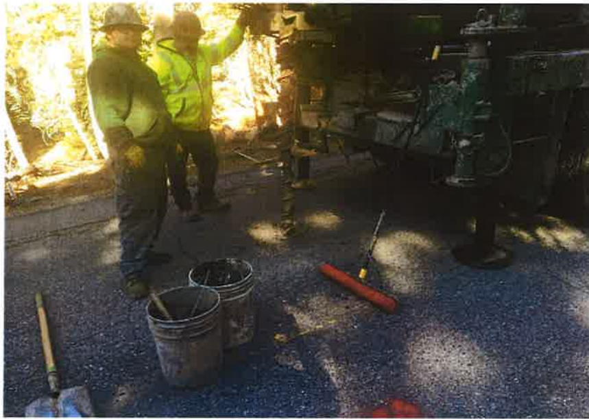
Photograph 37. Boring SW-B-37 during drilling.
