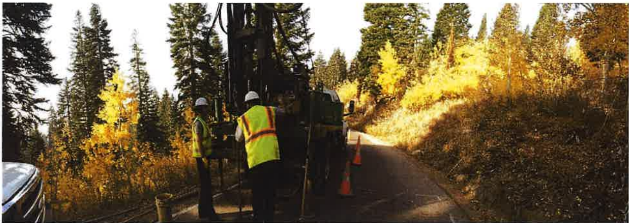
Photograph 52. Boring SW-B-44 during drilling.
