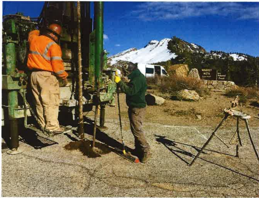
Photograph 1 - boring SW-B-01 during drilling.
