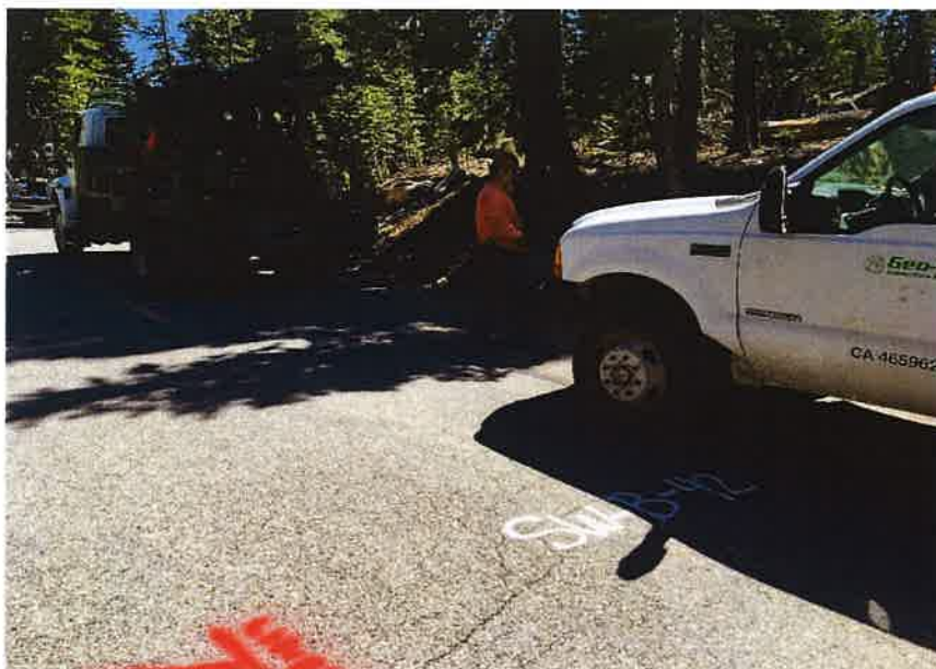
Photograph 42. Boring SW-B-42 after drilling.
