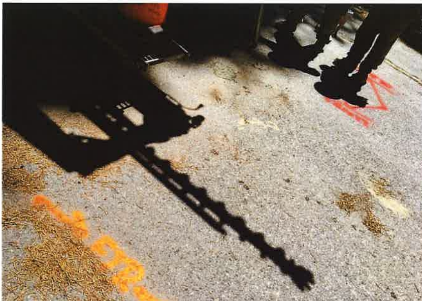
Photograph 38. Boring SW-B-38 after drilling.
