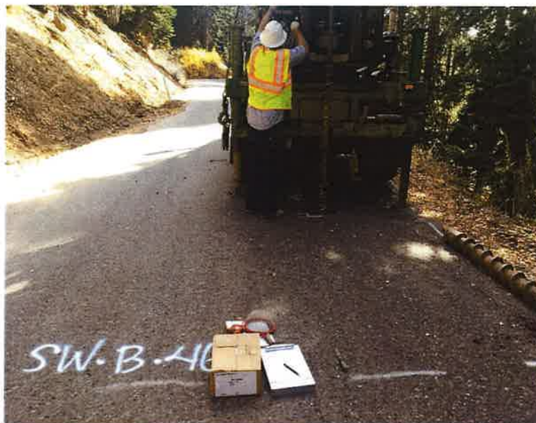
Photograph 54. Boring SW-B-46 during drilling.
