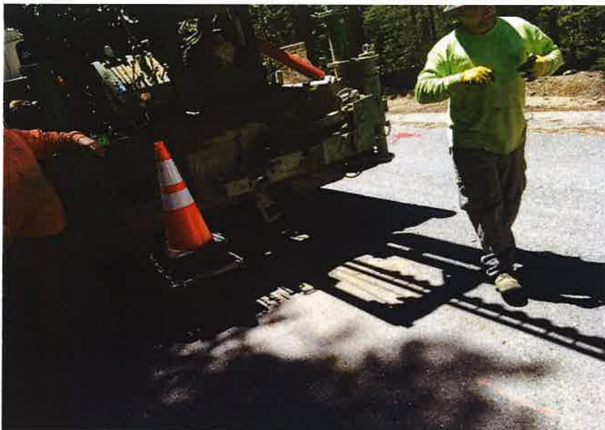
Photograph 36. Boring SW-B-36 during drilling.
