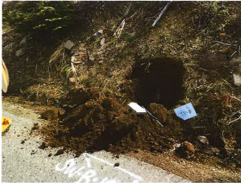
Photograph 49. Test Pit TP-6 during excavation.
