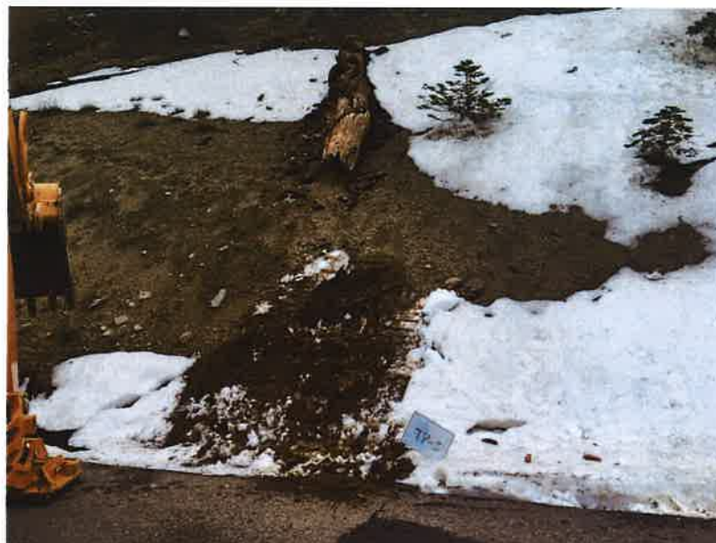
Photograph 46. Test Pit TP-3 during excavation.
