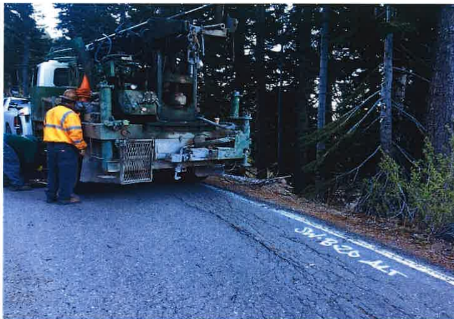
Photograph 20. Boring SW-B-20 before drilling.
