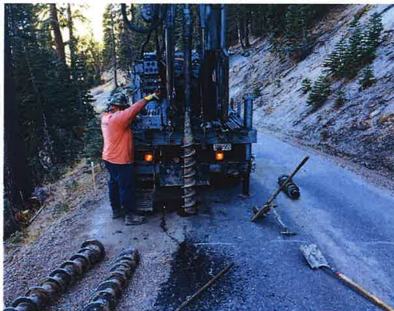
Photograph 56. Boring SW-B-48 during drilling.
