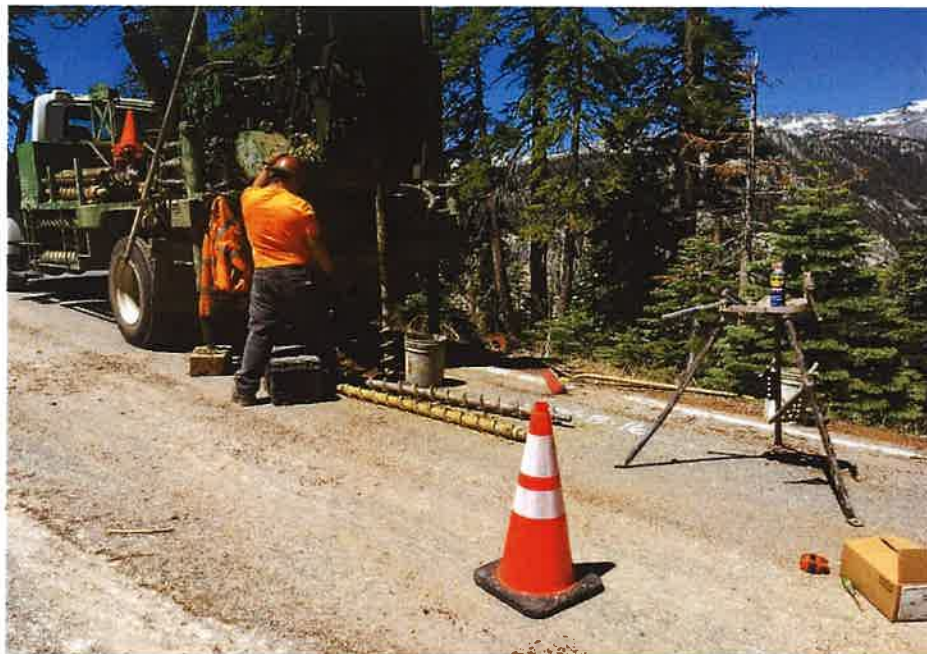
Photograph 16. Boring SW-B-16 during drilling.
