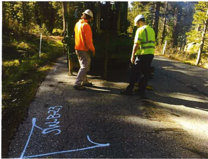
Photograph 23. Boring SW-B-23 during drilling.
