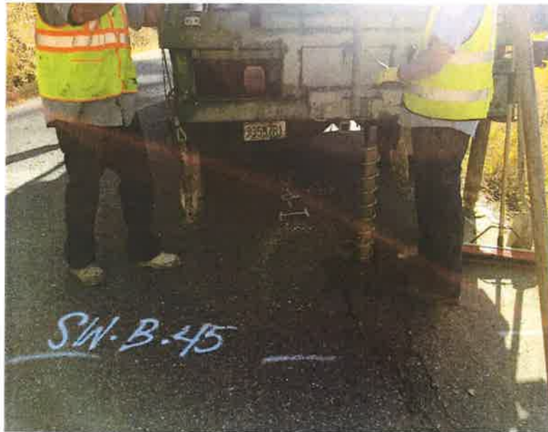
Photograph 53. Boring SW-B-45 during drilling.
