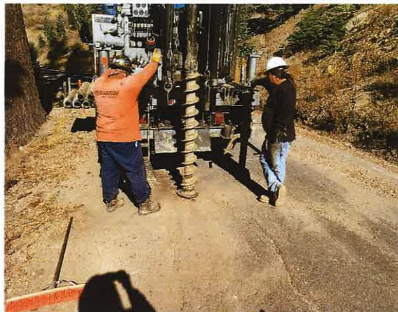
Photograph 58. Boring SW-B-50 during drilling.
