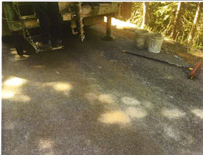
Photograph 21. Boring SW-B-21 before drilling.
