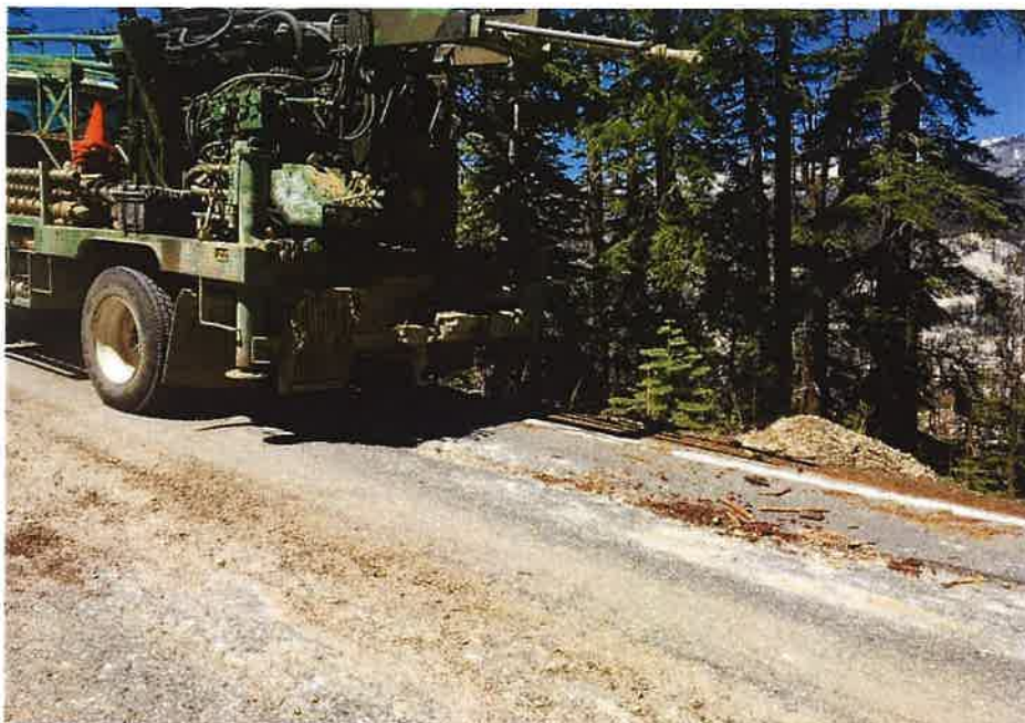
Photograph 8. Boring SW-B-08 during drilling.
