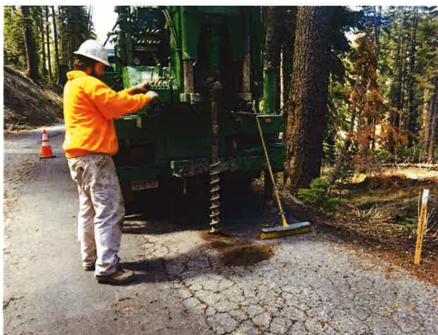
Photograph 26. Boring SW-B-26 during drilling.
