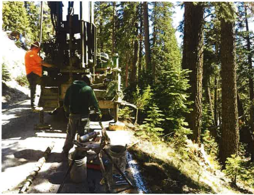
Photograph 11. Boring SW-B-11 during drilling.
