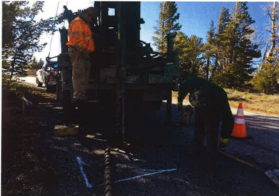
Photograph 2 - boring SW-B-02 during drilling.
