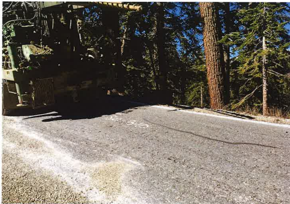
Photograph 10. Boring SW-B-10 before drilling.
