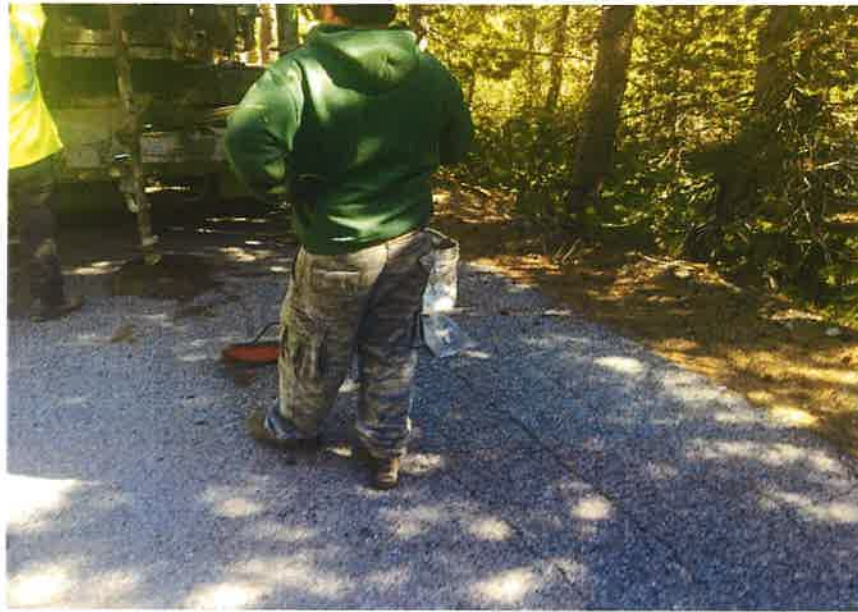
Photograph 33. Boring SW-B-33 during drilling.
