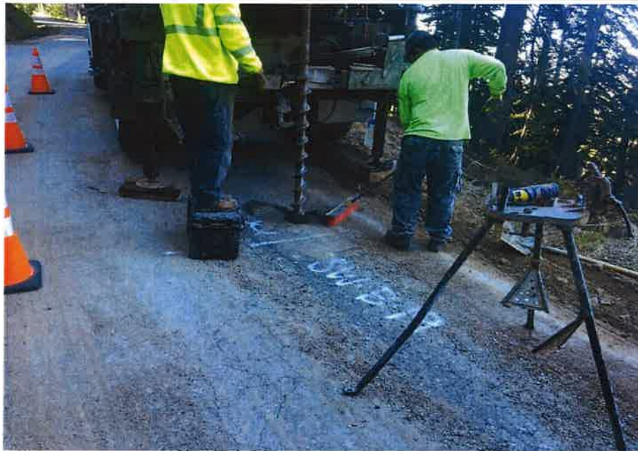
Photograph 19. Boring SW-B-19 during drilling.
