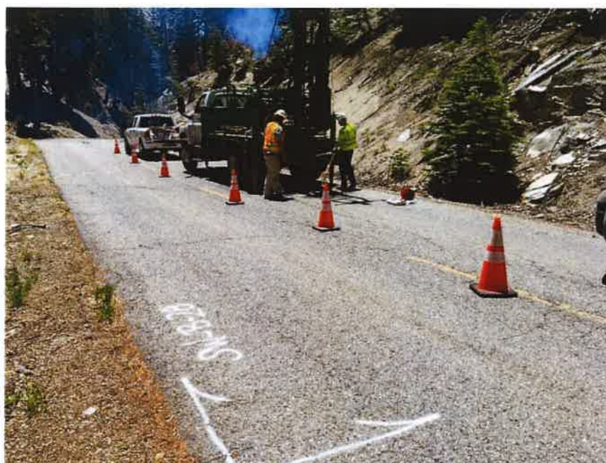
Photograph 28. Boring SW-B-28 during drilling.
