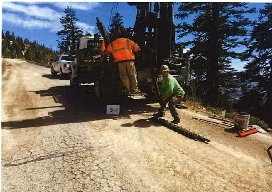
Photograph 4. Boring SW-B-04 during drilling.
