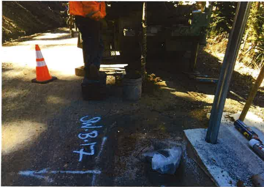
Photograph 17. Boring SW-B-17 during drilling.
