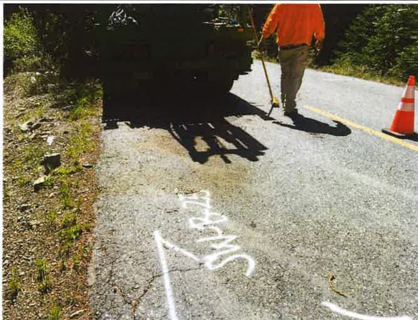
Photograph 25. Boring SW-B-25 during drilling.
