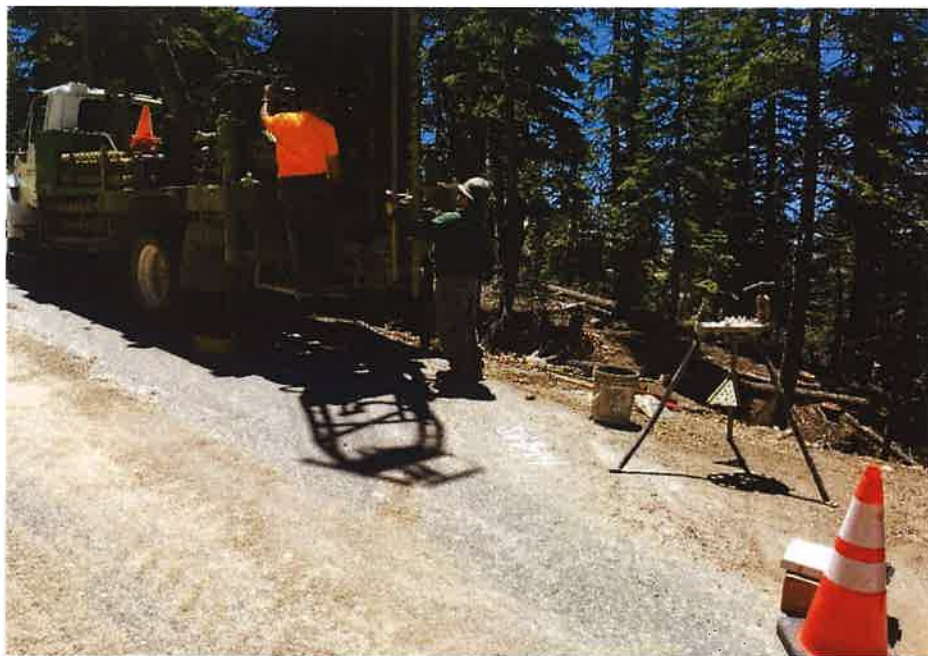
Photograph 14. Boring SW-B-14 before drilling.
