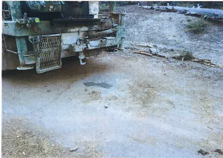
Photograph 43. Boring SW-B-43 during drilling.
