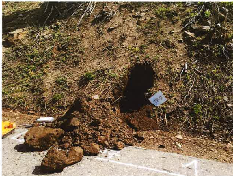
Photograph 50. Test Pit TP-7 during excavation.
