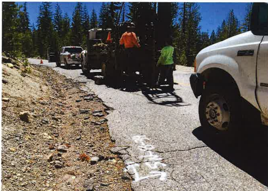
Photograph 34. Boring SW-B-34 during drilling.
