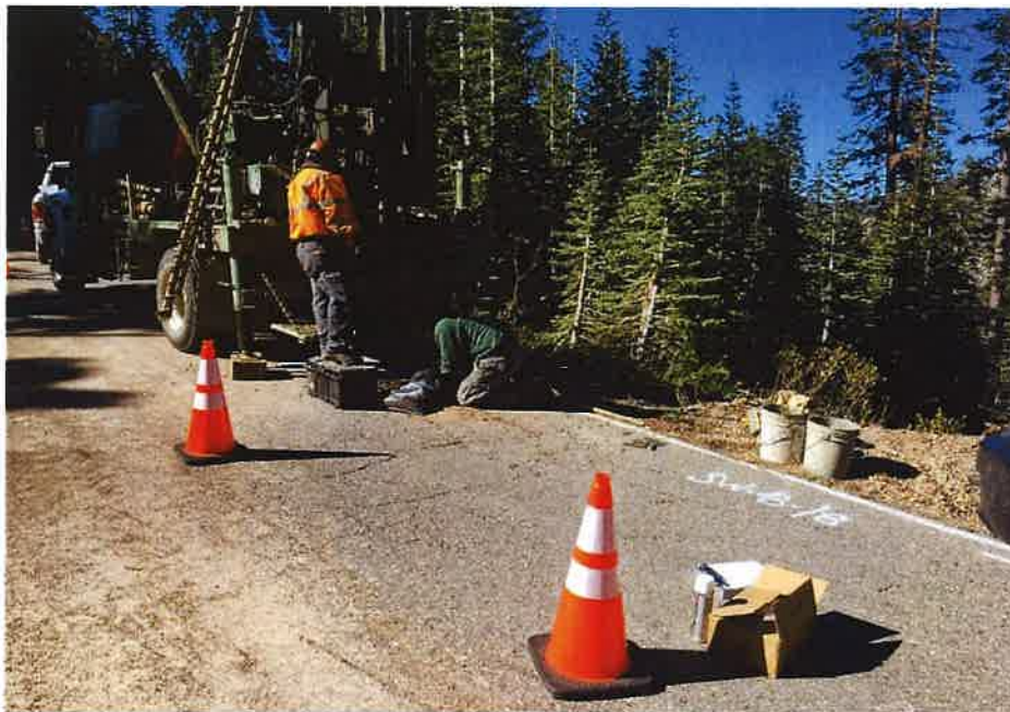
Photograph 18. Boring SW-B-18 during drilling.
