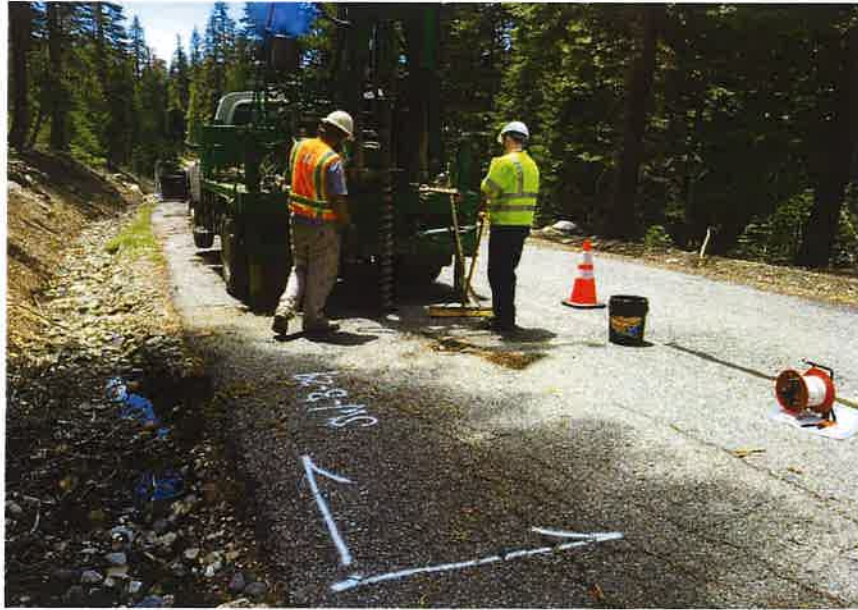
Photograph 29. Boring SW-B-29 during drilling.
