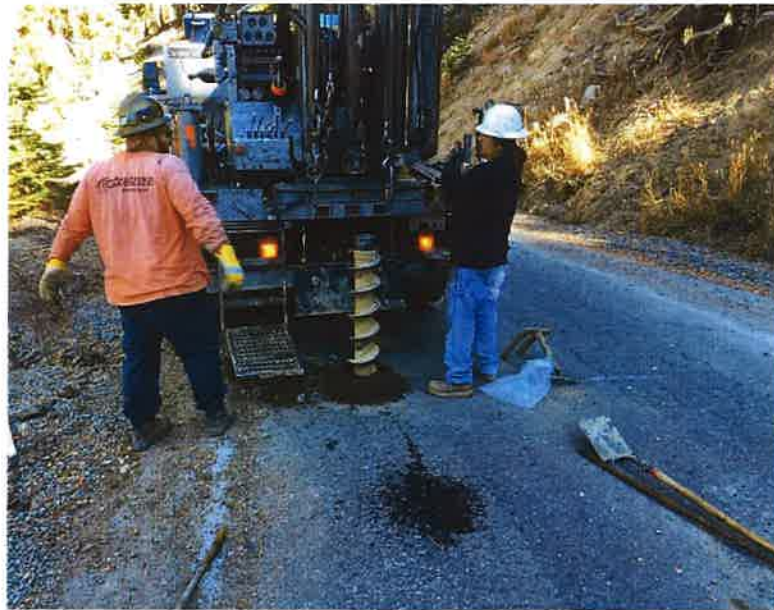
Photograph 57. Boring SW-B-49 during drilling.
