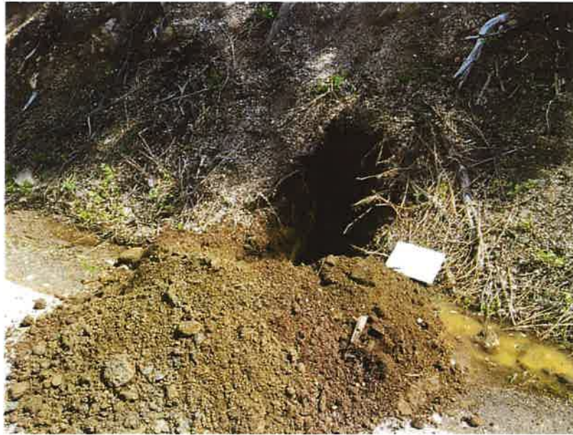
Photograph 51. Test Pit TP-8 during excavation.
