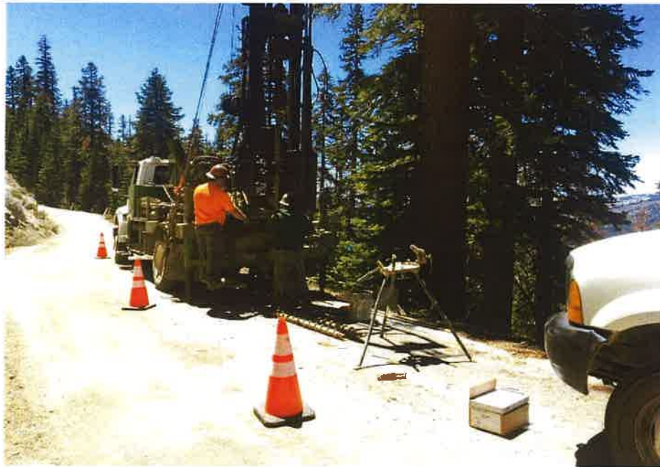
Photograph 15. Boring SW-B-15 during drilling.
