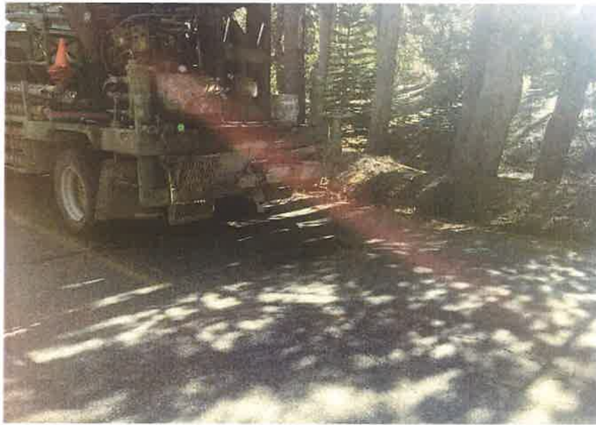
Photograph 35. Boring SW-B-35 during drilling.
