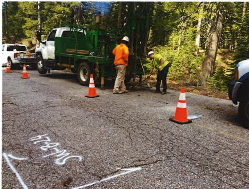
Photograph 24. Boring SW-B-24 during drilling.
