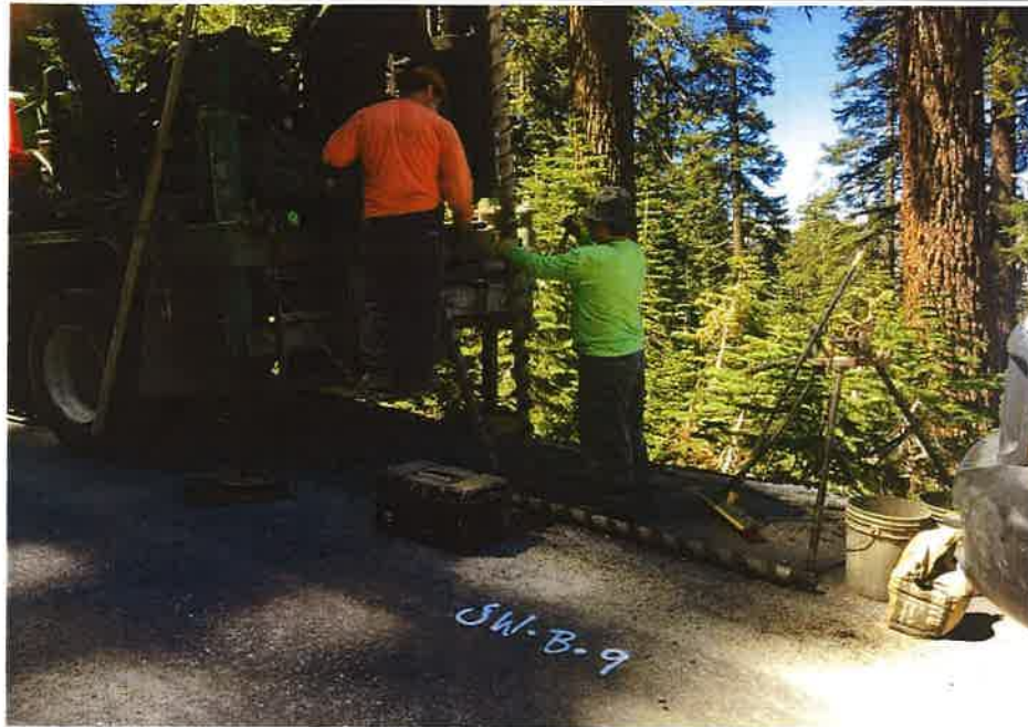
Photograph 9. Boring SW-B-09 during drilling.
