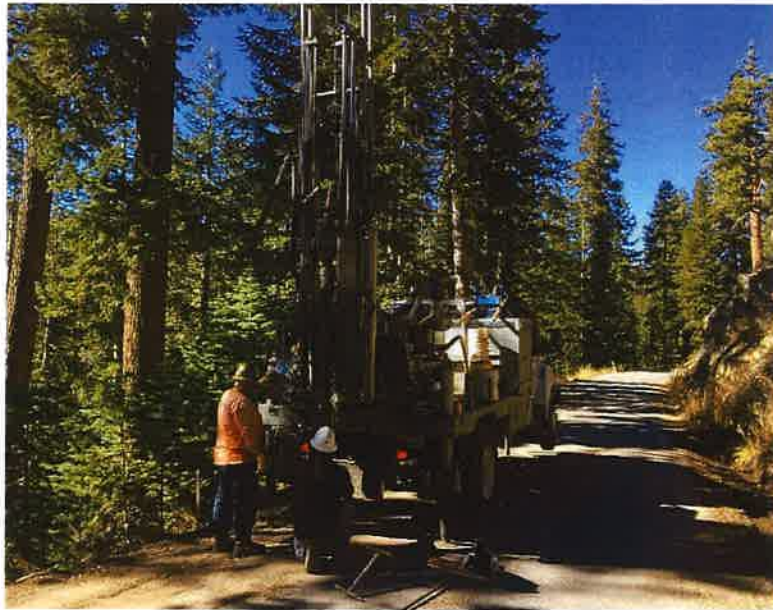
Photograph 59. Boring SW-B-51 during drilling.
