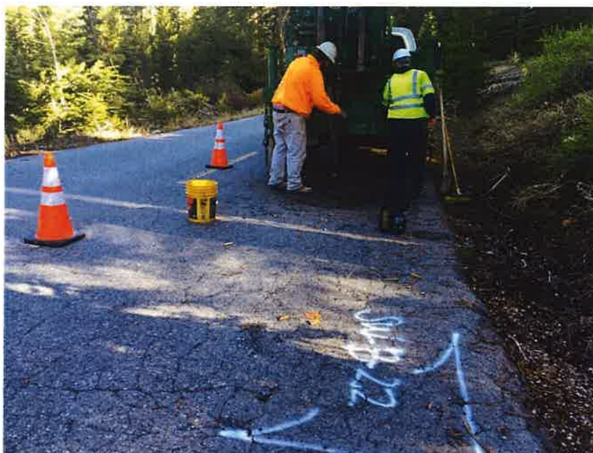
Photograph 22. Boring SW-B-22 during drilling.
