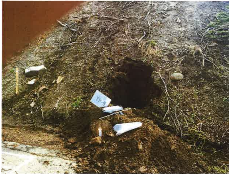
Photograph 47. Test Pit TP-4 during excavation.
