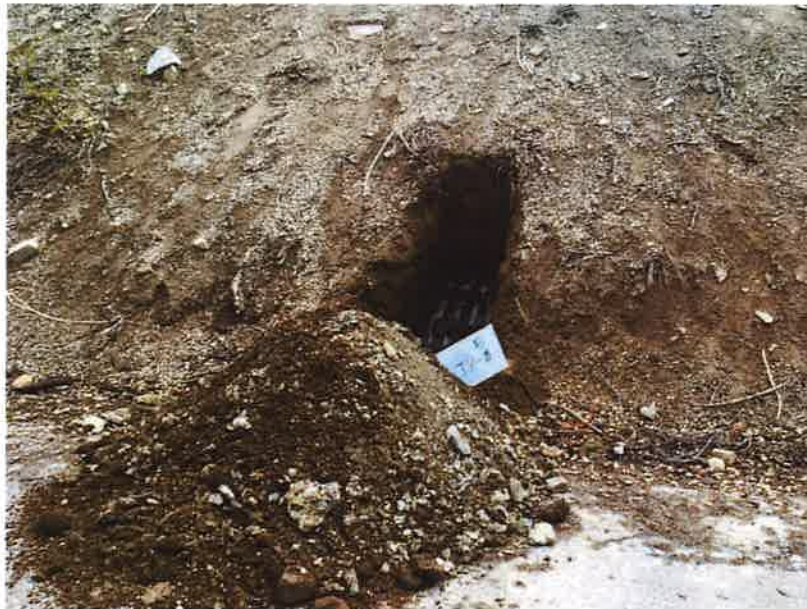
Photograph 48. Test Pit TP-5 during excavation.
