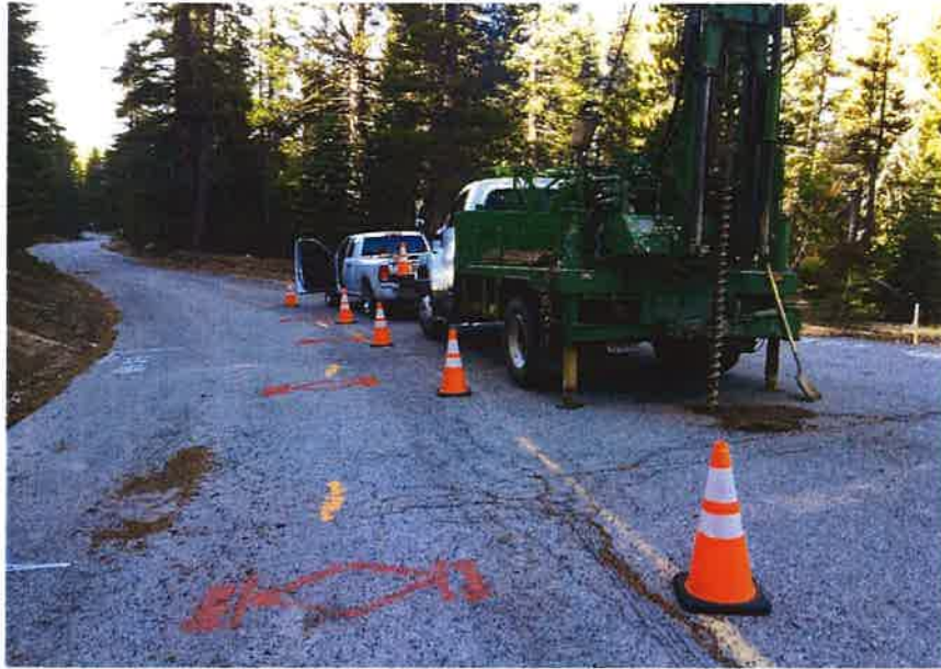
Photograph 31. Boring SW-B-31 during drilling.
