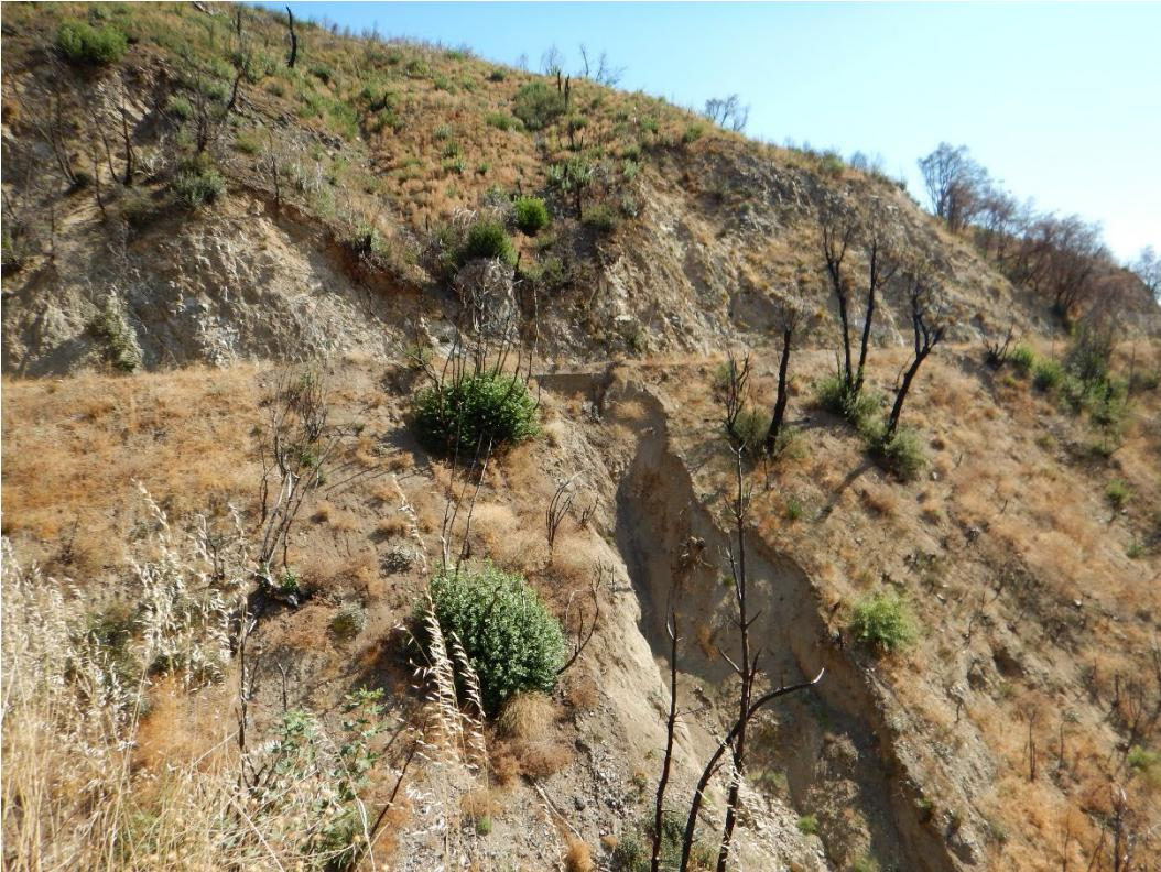
**Photo 17: Embankment failure**
