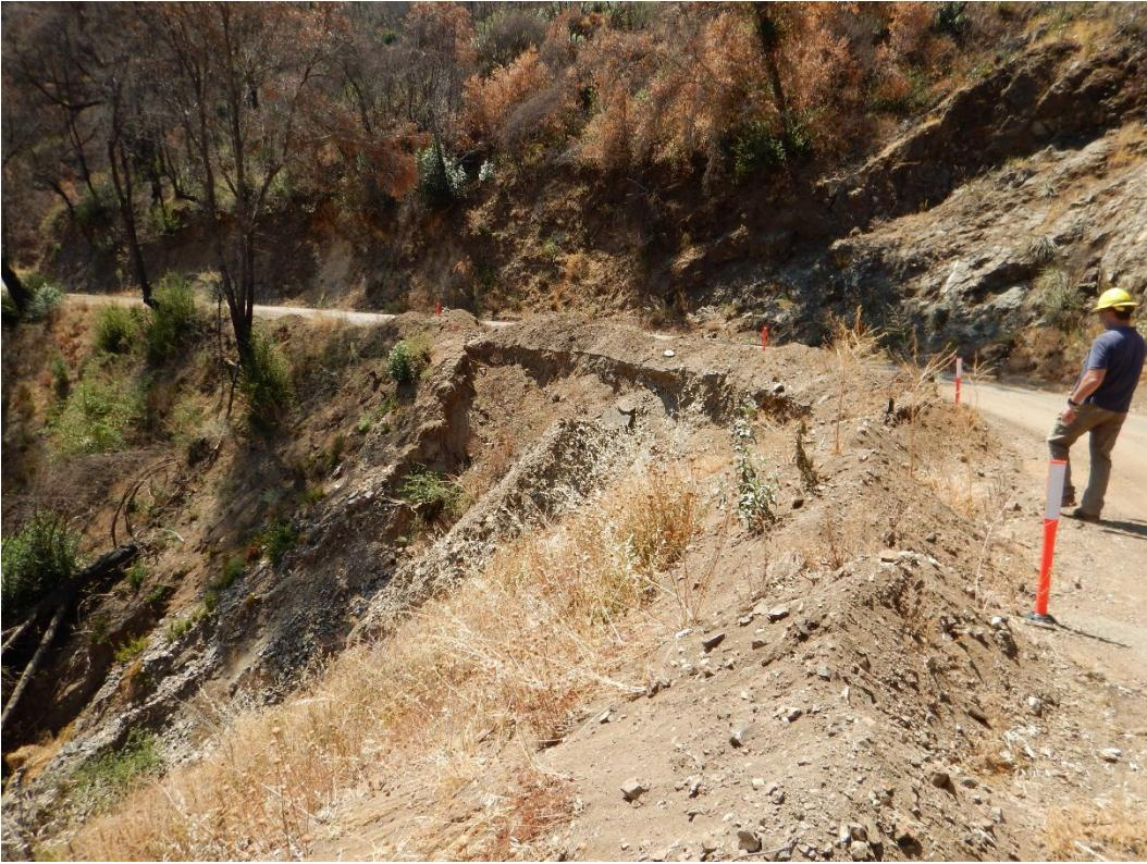
**Photo 11: Embankment failure looking up station**
