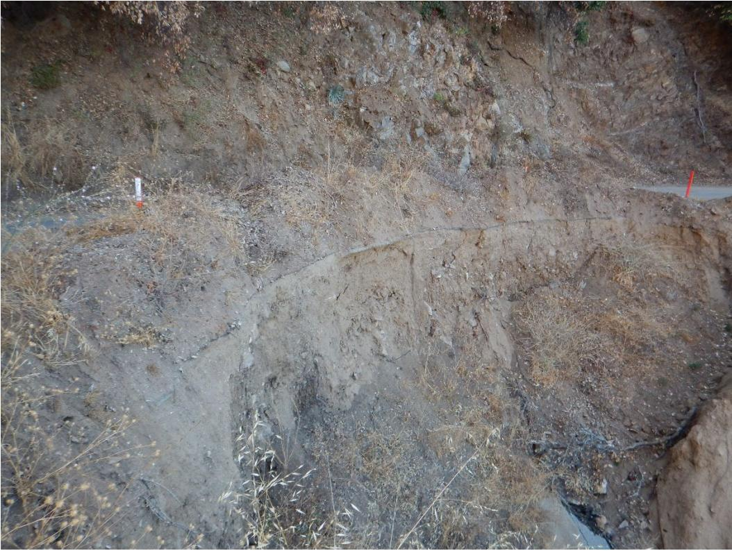
**Photo 21: Embankment failure / erosion**
