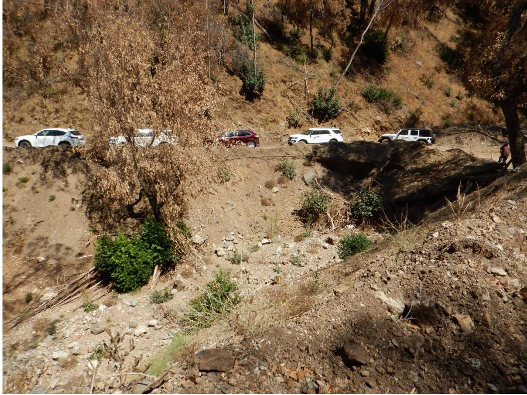
**Photo 7: Overall site with debris piled on shoulders, embankment erosion below red vehicle**
