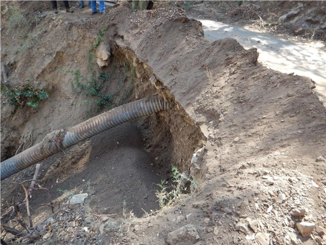
**Photo 13: Embankment failure around culvert**
