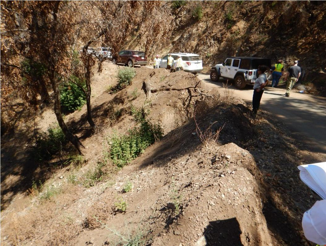
**Photo 6: Embankment erosion**
