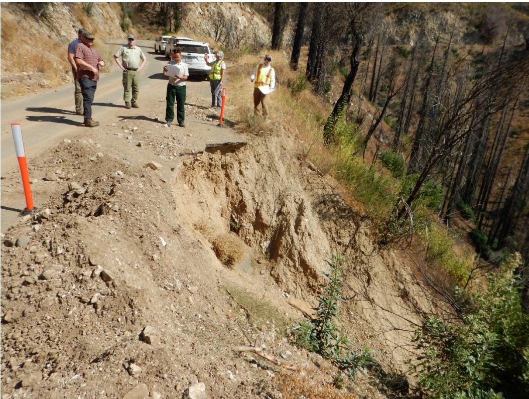
**Photo 19: Embankment failure**
