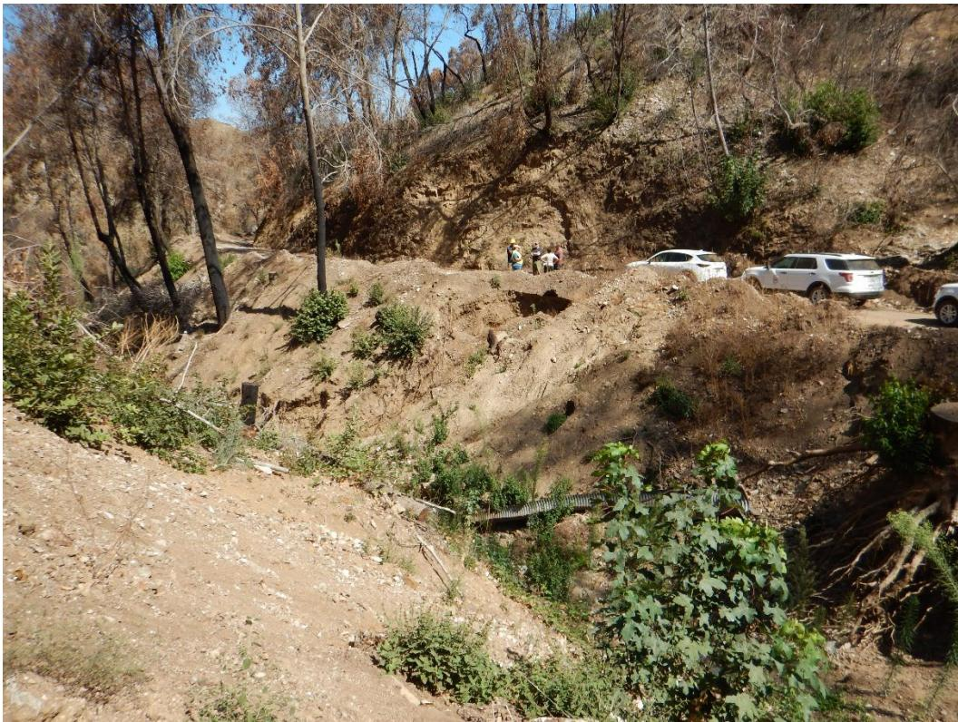
**Photo 16: Embankment failure due to scour and erosion in channel**
