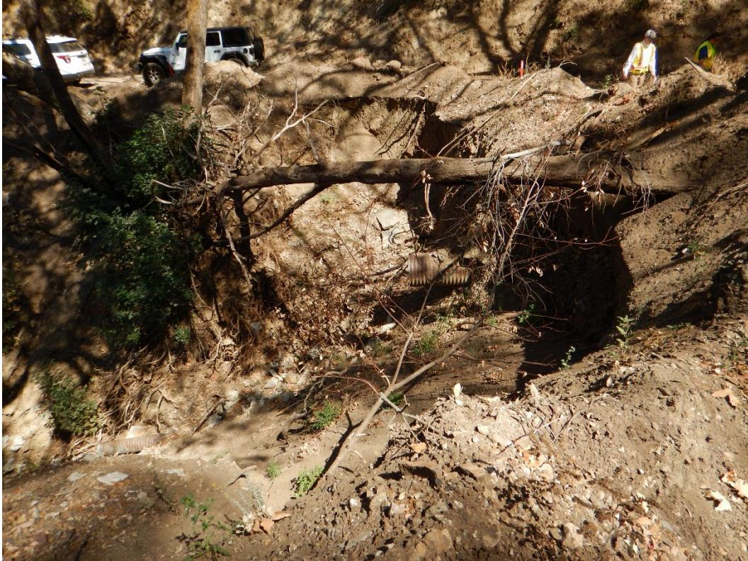
**Photo 3: Embankment erosion**
