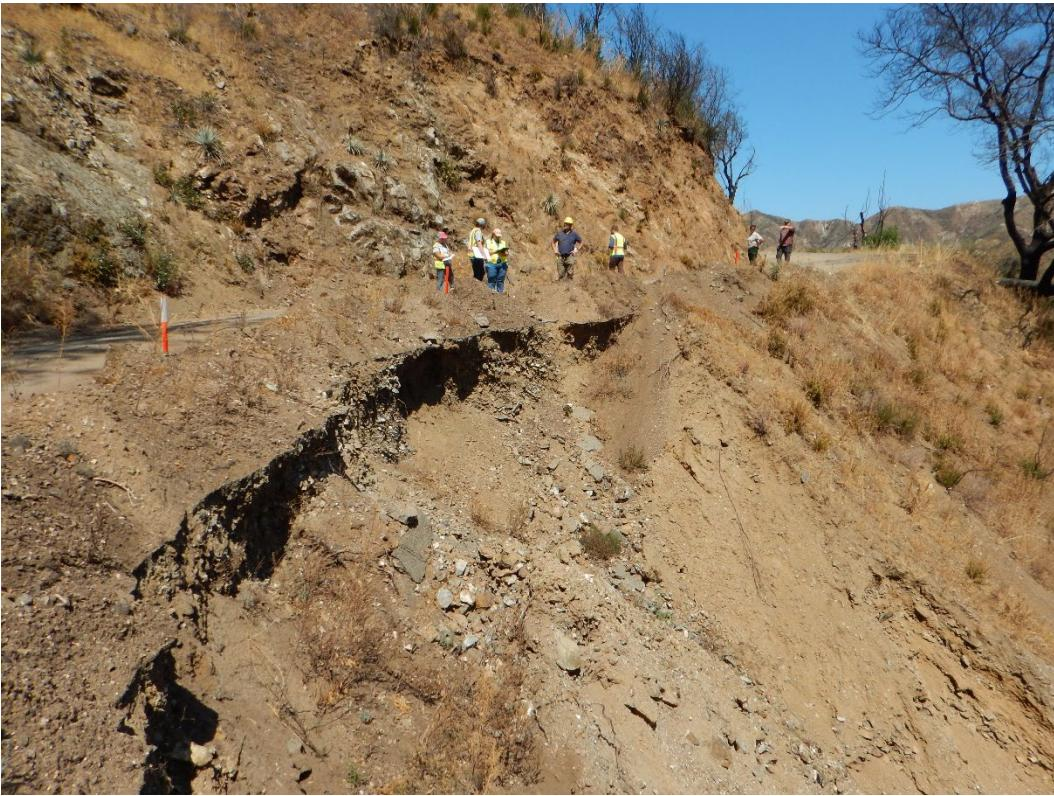
**Photo 12: Embankment failure looking downstation**
