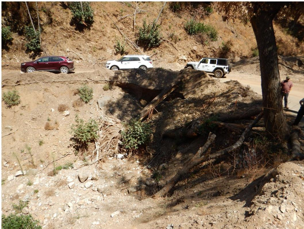
**Photo 8: Debris piles on shoulders and upstream channel, culvert outlet buried under debris**
