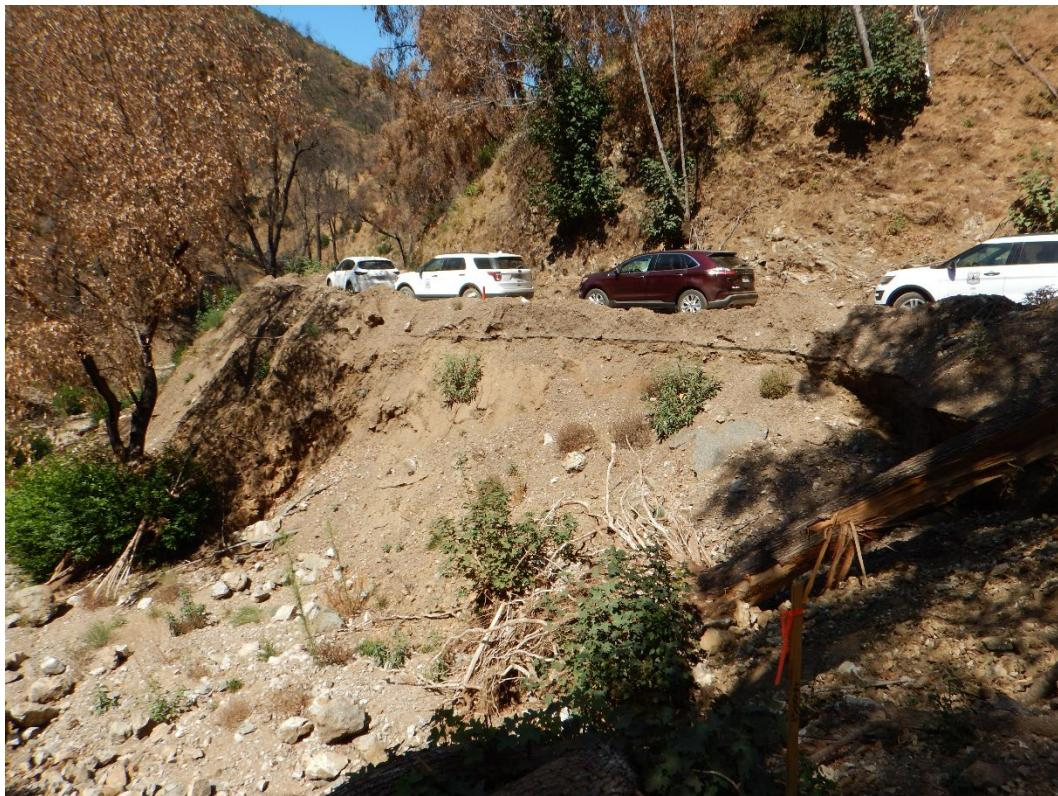
**Photo 10: Embankment failure due to scour and erosion of toe**
