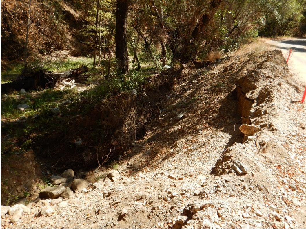
**Photo 1: Eroded embankment**
